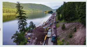
monitoring, PTZ cameras, and driveway-automated devices, were used to minimize wait times for the public traveling through the project area. The corridor was paved with plant mix asphalt and finished with chip and fog seal.
